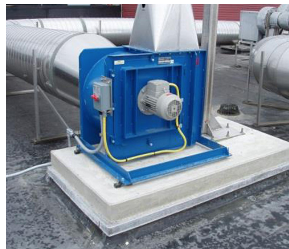
Fan placed on the roof.
