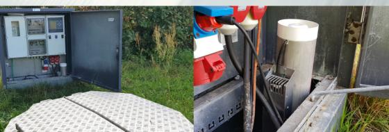
The HS Purifier is connected to a 230V power supply and is mounted vertical in an  $\emptyset$ II0 PVC tube with the ventilator on top.
